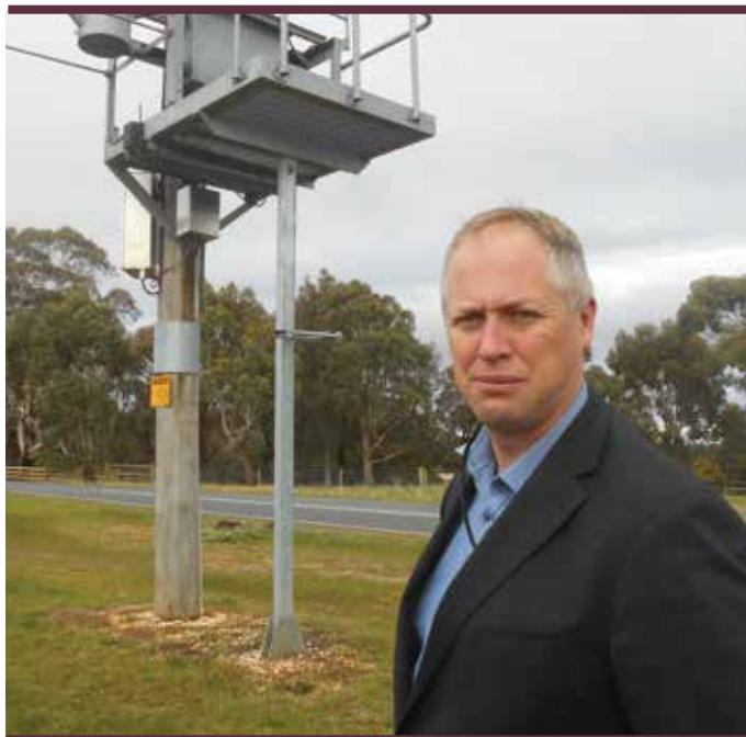
Powercor's Richard Scholten on Durham Lead Road near where the battery power back-up unit will be connected to existing transmission lines.
