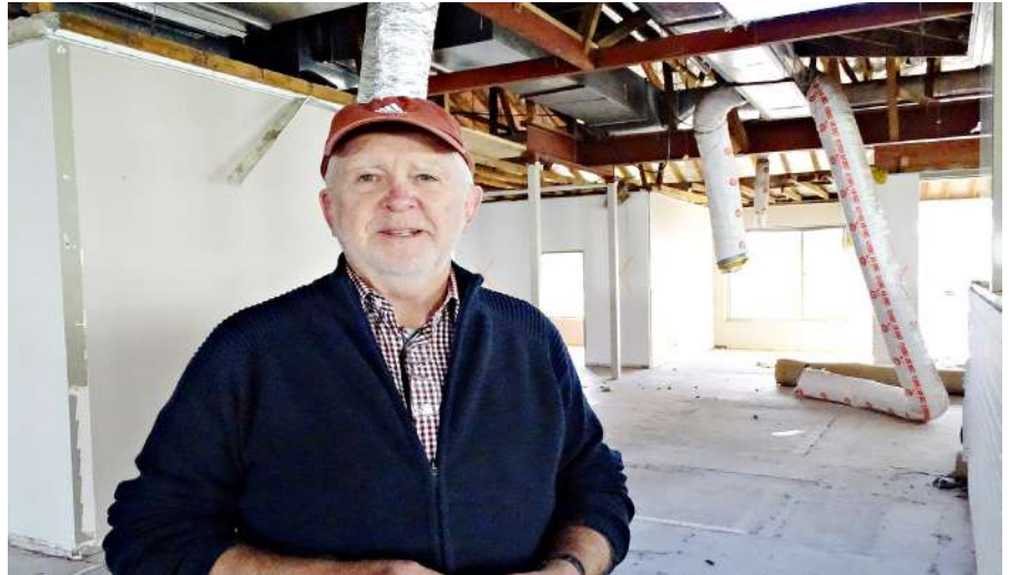
Gerard Ballantyne inspects the demolition work inside Village Place.
