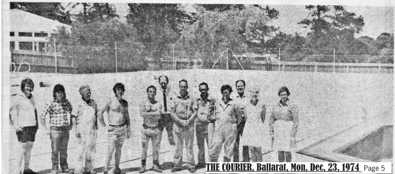
Photograph of the pool opening (Ballarat Courier of 23 December 1974) showing Committee members and volunteers standing in the completed pool.
